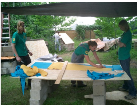
cutting roof fabric
